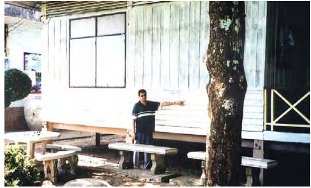
Showing the level the water reached at the last flood
